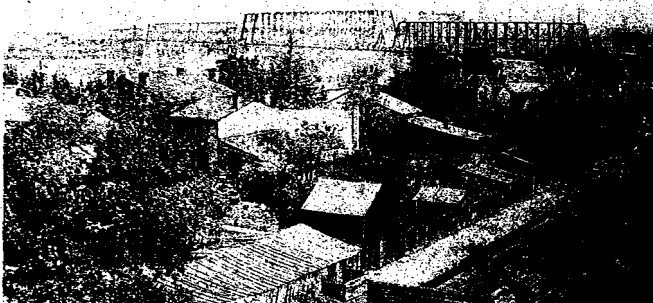
North-East From Roof
