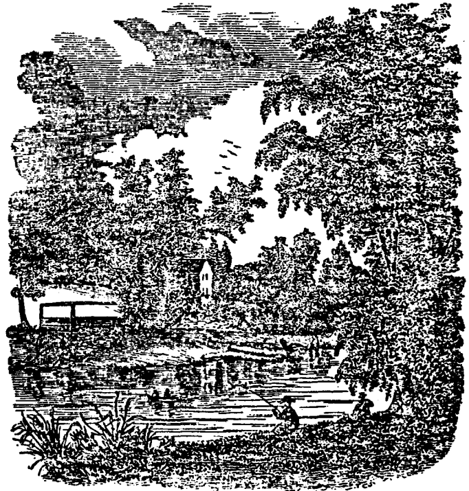
VIEW OF BANK LICK, KENTON CO., KY.
