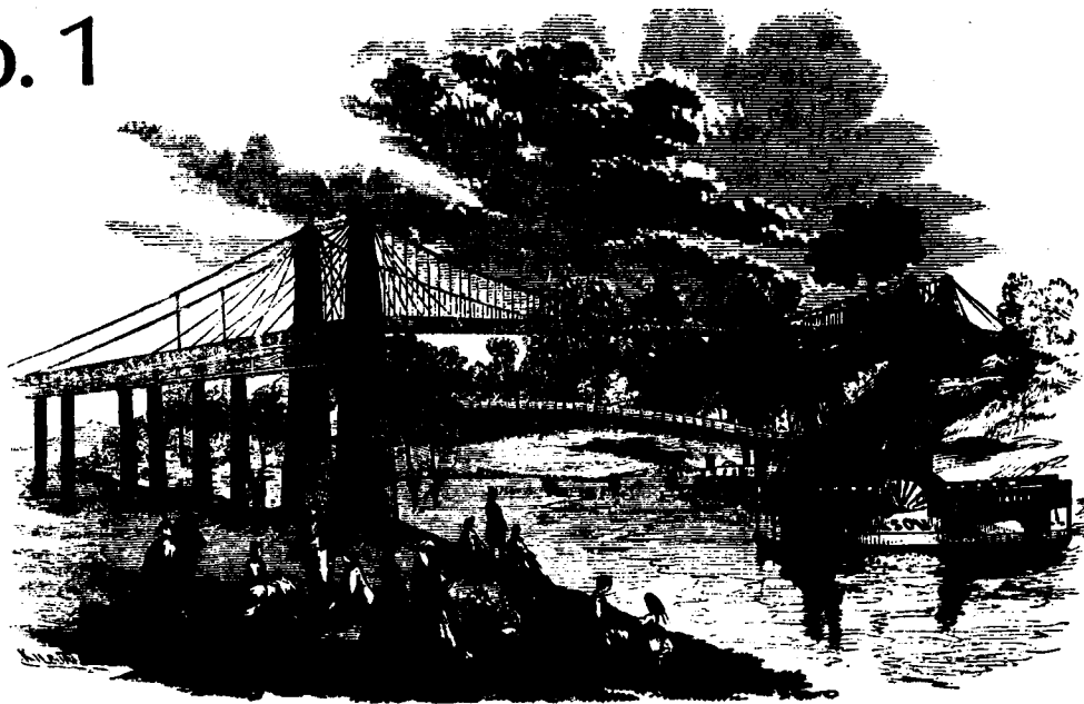
SUSPENSION BRIDGE OVER THE LICKING RIVER.
